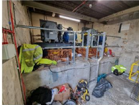
New lift motor platform edge protection
