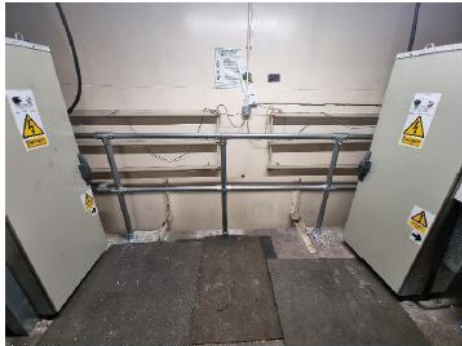
New lift motor platform rear edge protection
