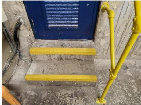
New handrail and colour contrast nosing's
